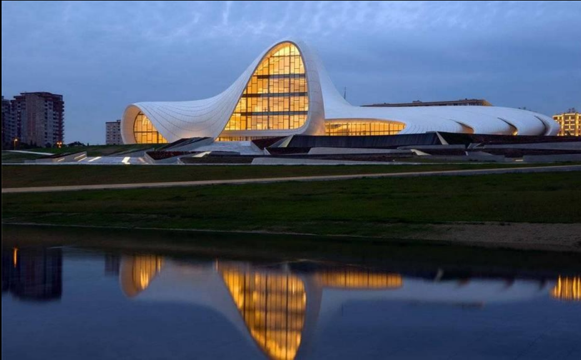
Heydar Alyev Cultural Center. A: Zaha Hadid Architects E: Werner Sobek Stuttgart
